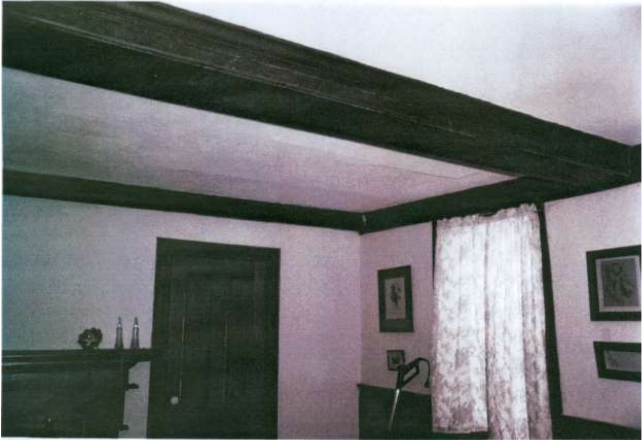
Southwest (dining) room, showing ceiling framing with cased beams and cornice detail. Photographer Mrs. Richard Anderson, 1982
