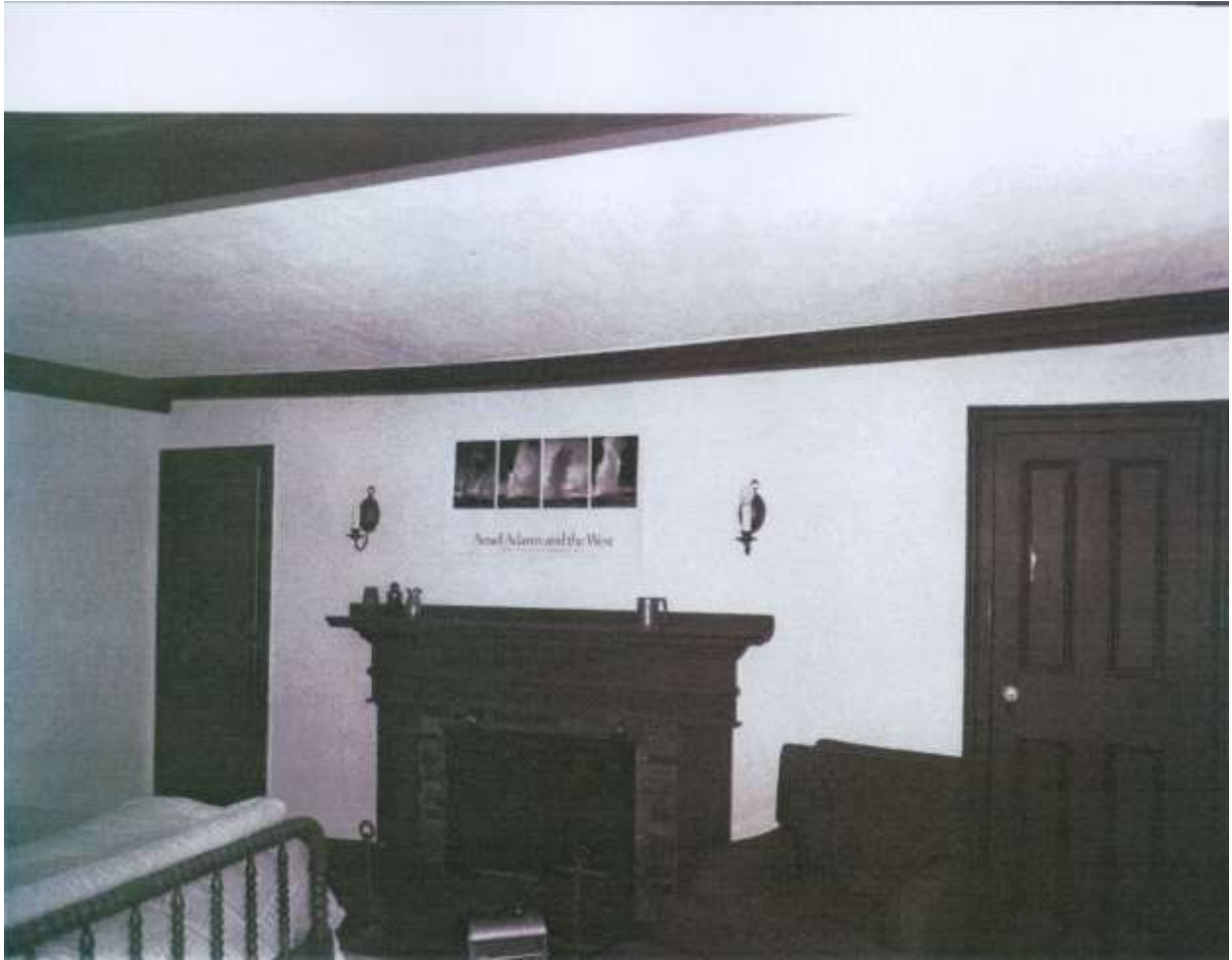
Southwest chamber, showing one story mantel-piece, two-panel close door, four-panel door into upstairs south hall, cased summer beams. Photographer Mrs. Richard Anderson, 1982
