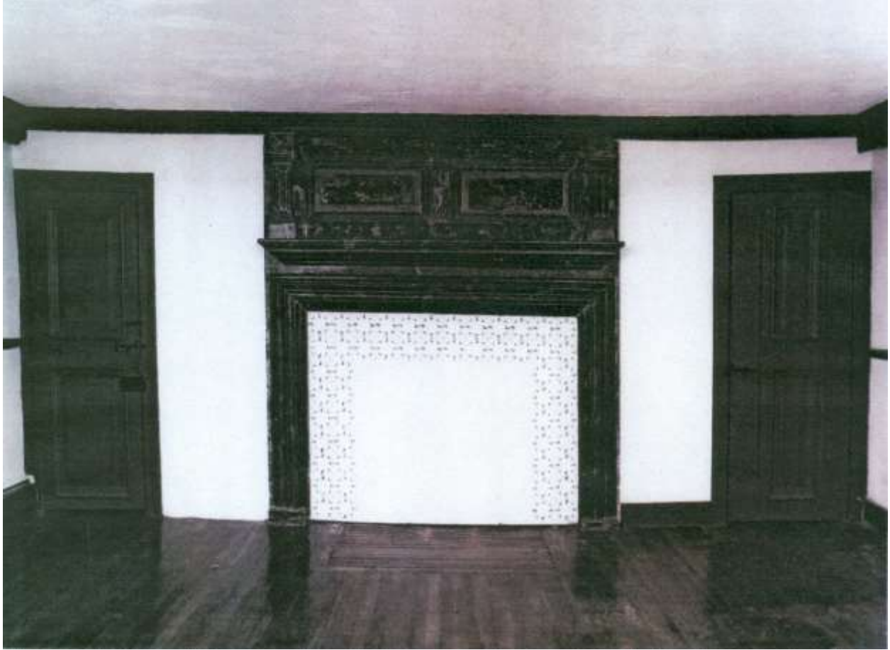
Northwest chamber (Lafayette Room) showing mantelpiece with bolection paneling, restored marbleizing, two panel doors, still sainted and to be restored. Photographer: John Shotwell, 1982
