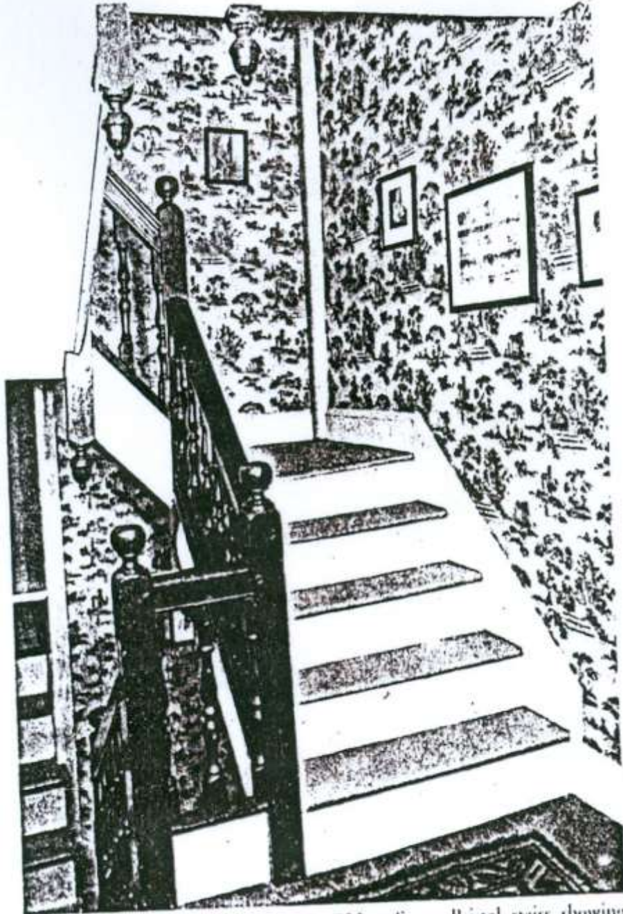
PLATE 20. Joseph Reynolds House, 956 Hope Street, Bristol, stairs, showing half balusters abutting the posts, and the hand rail moulded on the outer edge only.
