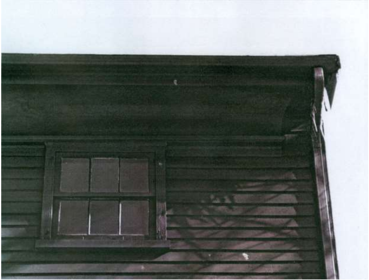
Joseph Reynolds house, west front detail showing cove cornice and old window. Photographer John Shotwell
