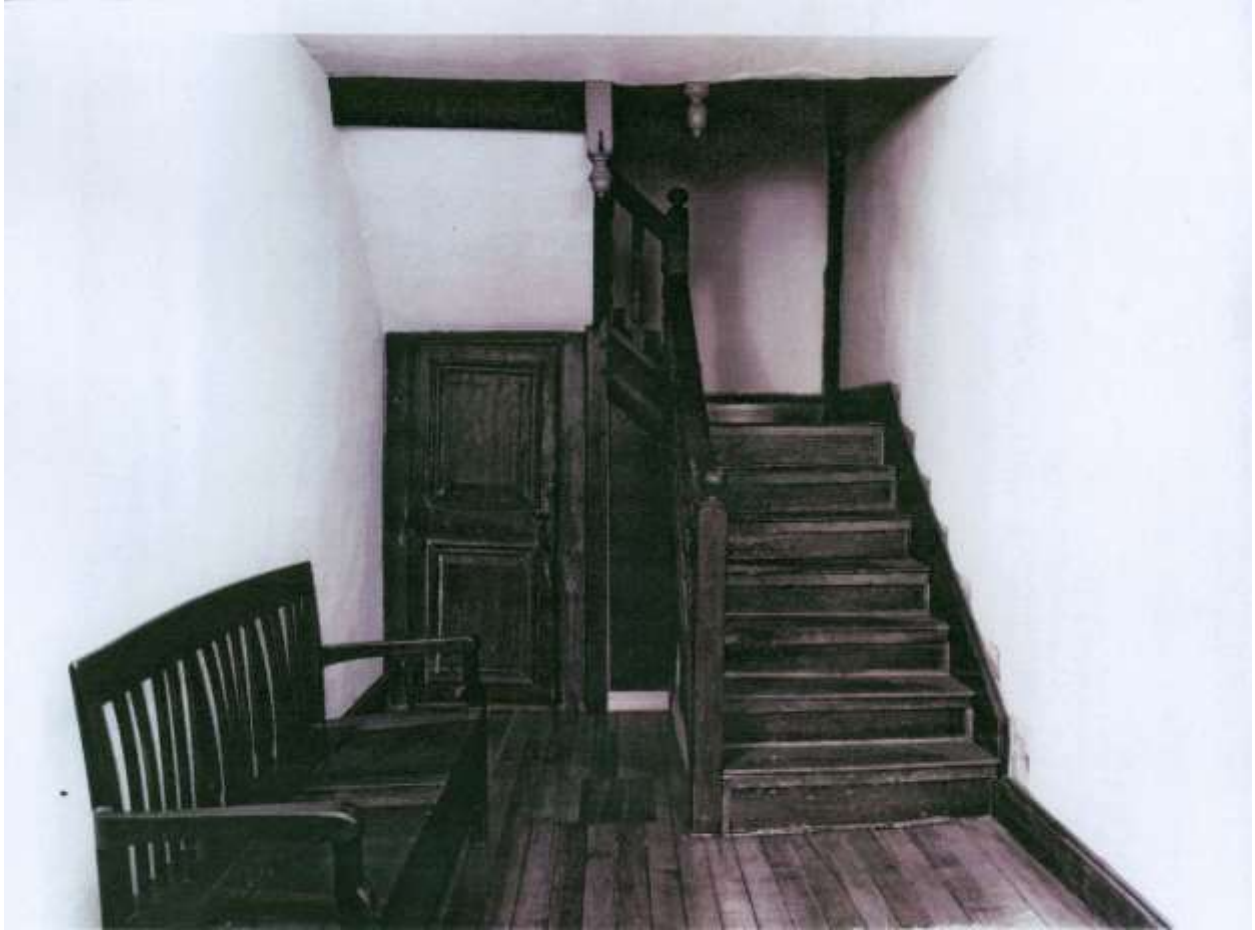
Stairway, first floor hall, showing two-panel door into rear room. Painted riser line showing above riser board. Photographer: John Shotwell, 1982
