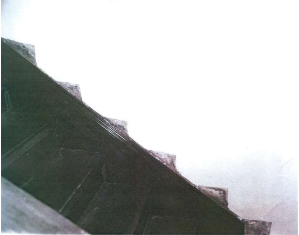
Stair, second to third story, showing old painting defining riser behind the later stair casing. Photographer Mrs. Richard Anderson, 1982
